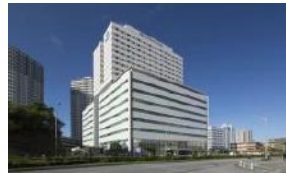
Naha Shin-Toshin Center Building
