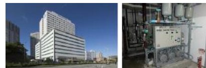
Naha Shin-Toshin Center Building.
