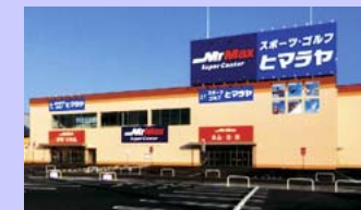
Okayama Kume Retail Facility
