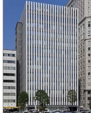
ORE Sapporo Building
