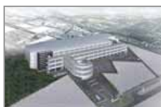
(Provisional) Yokohama Machida IC Logistics Center
